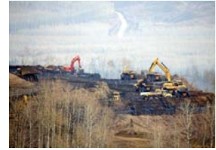
Contractors excavate soil to prepare for Site C construction.
