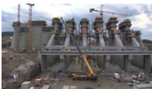
Muskrat Falls Hydro Power Project Under Construction.
